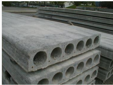
Hollow Core Precast Slab
